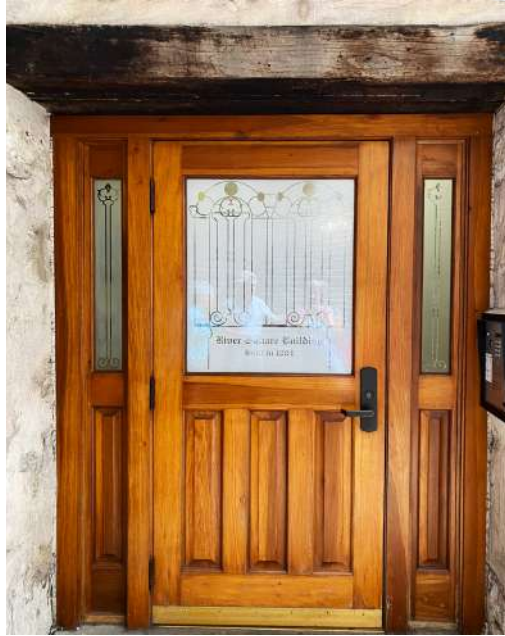
Secured Private Entry to Building
