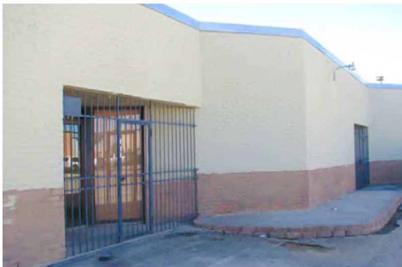
Secured front entrance.
