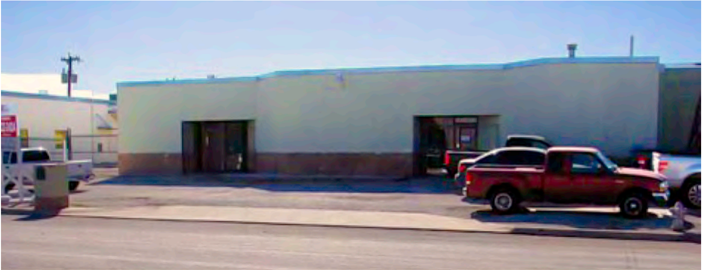
Front of building.
